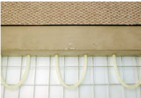
1A. PEX tubing in slab
