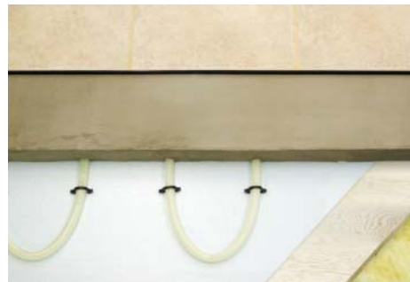
3A. Light concrete is poured onto suspended wood sub floor
