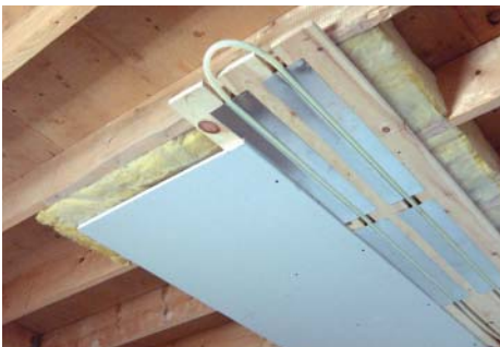
4. Aluminum plates on Ceiling
